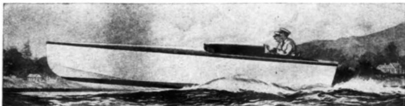
Instead of being attached to the stern in the conventional manner, the outboard motor which propels this boat is installed through a well in the hull.
