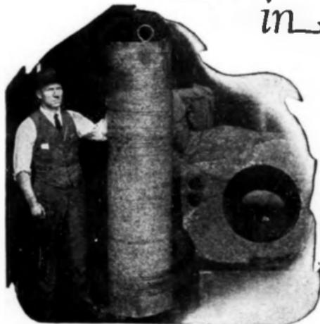
How would you like to bite this six-foot cylinder out of a block of solid granite? A new rotary core drill cut this tube out of the granite slab in a few hours.
