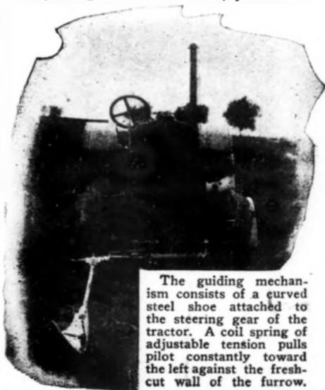
The guiding mechanism consists of a curved steel shoe attached to the steering gear of the tractor. A coil spring of adjustable tension pulls pilot constantly toward the left against the fresh-cut wall of the furrow.
