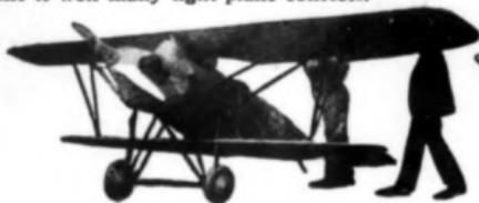
The Myers Midget can do 100 miles an hour with ease. It is a single seater with a two-cylinder engine. The span is only 16 feet.
