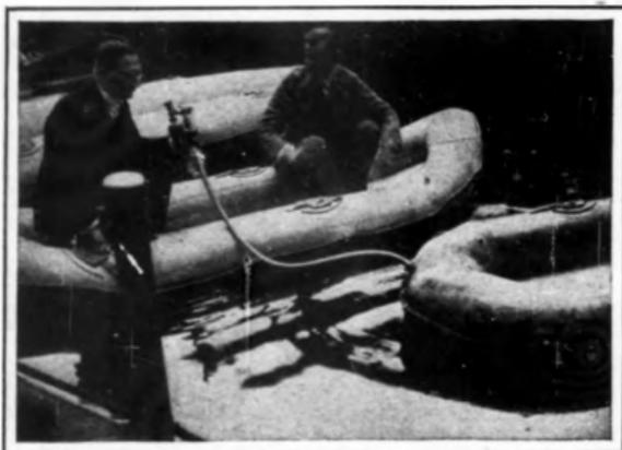
These rubber life rafts are shown being inflated from a tube of compressed air. Note leather oarlocks.
