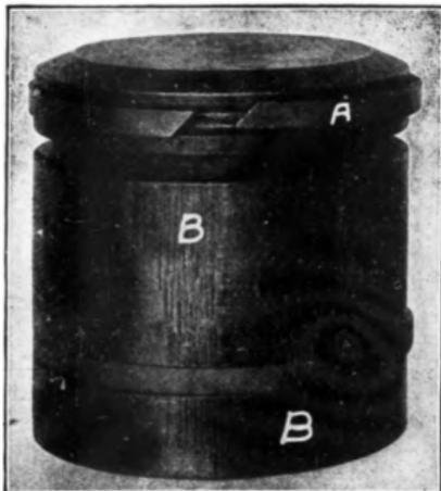
Overheating has ruined this piston. Note warping of ring at A and scoring of piston at B B.
