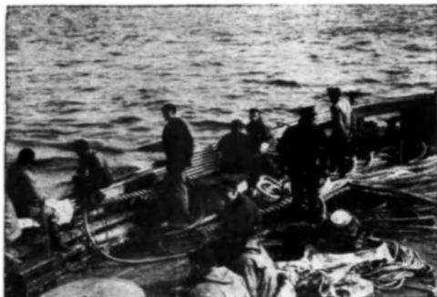
The stern of the U. S. S. Falcon, Uncle Sam's salvage ship. Here the oil stored in the S-4 is being transferred to tanks aboard the Falcon, through the salvage hose shown going over the rail on which the sailor is sitting.
