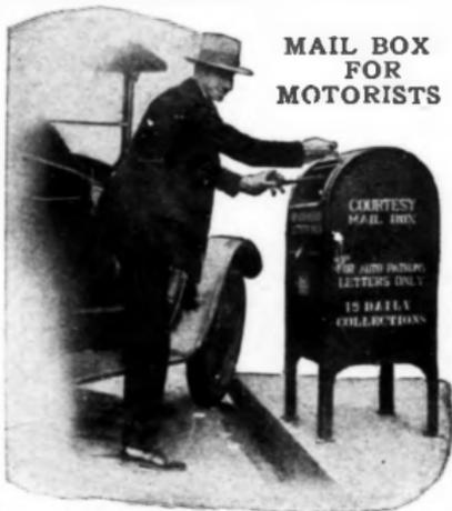
Mail boxes equipped with an extension lever and placed close to the curb so that motorists can drive up to the sidewalk and mail letters from their cars have been installed in Sacramento and Oakland, Cal. They are proving very convenient for motorists.
